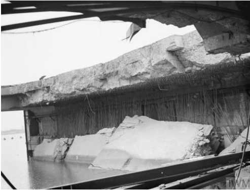
Damage to the E-Boat Pens at Le Havre after the strike by 617SQN using Tallboys on 14 June 1944. (IWM)
