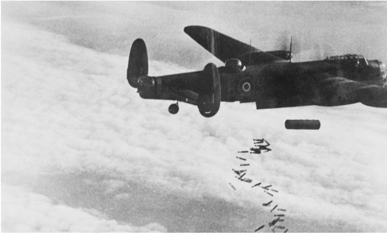
A Bomber Command Lancaster drops its bomb load of a 4,000lb 'cookie' and smaller incendiary bombs at high altitude over a target. This bomb load was the standard load employed by Bomber Command Lancasters through the war with the large 'cookie' designed to achieve significant blast damage and the smaller incendiary bombs designed to create fires. (AWM)
